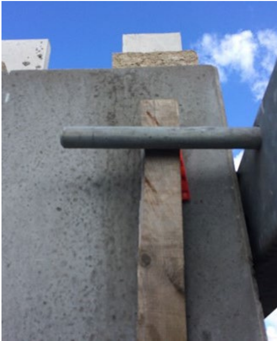
The mandrel and wooden wedge secure the element.
