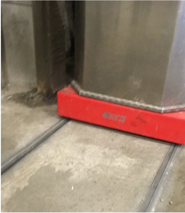
SP-SRS rails at Thomas Beton, Uddevalla, Sweden
