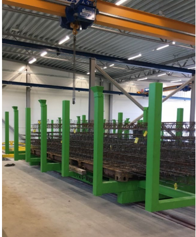
Racks placed on wagen
