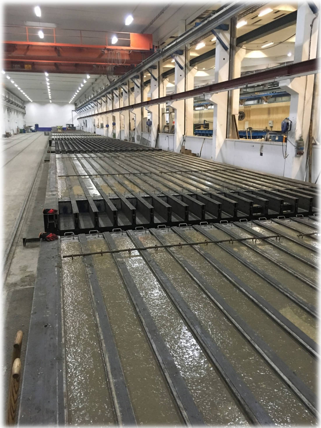
Image: Reinforced concrete pile production Sweden (Skanska AB)
