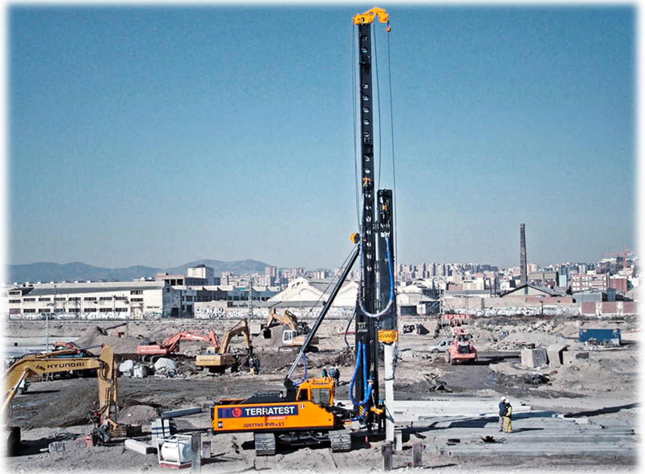
Picture: Site installation of precast piles. (PAA-Kazakhstan)
