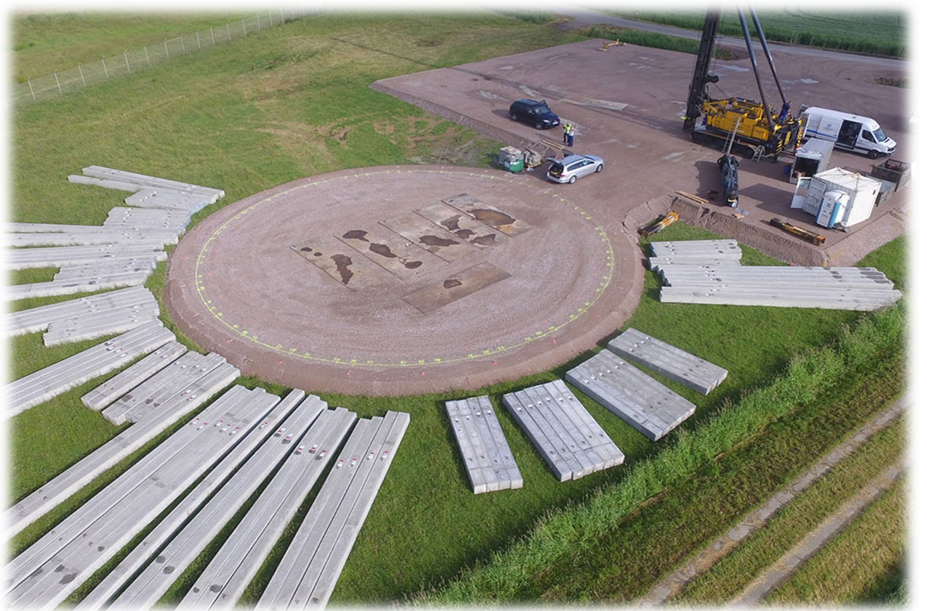
Picture: Precast piles ready for installation wind mill (CP-Germany)
